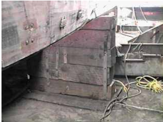
Bilge blocks supporting a vessel on a drydock.
