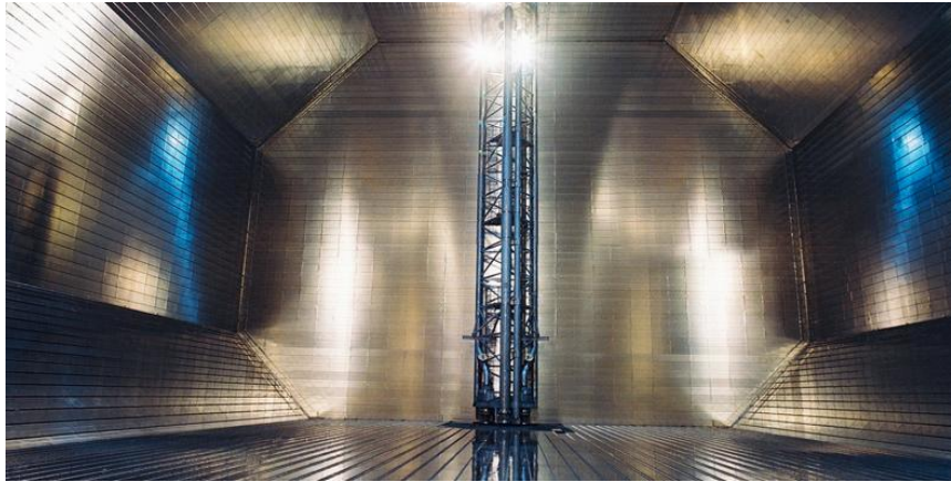
Image 3 Inside a GTT No96 tank
