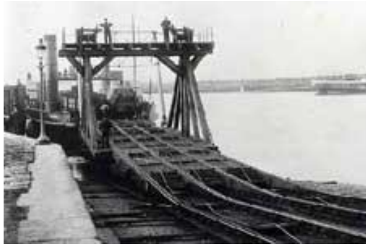
(Bouch's ferry design. Note the adjustable ramp)
