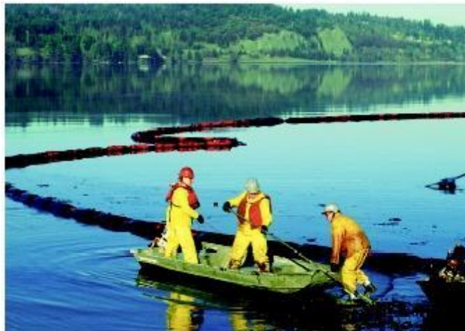
Workers clean up an oil refinery spill that polluted Anacortes Bay, Washington. The floating ring of absorbent pads trailing behind the boat is being used to contain some of the oil that has spilled.
