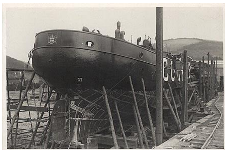
Lightship under construction
