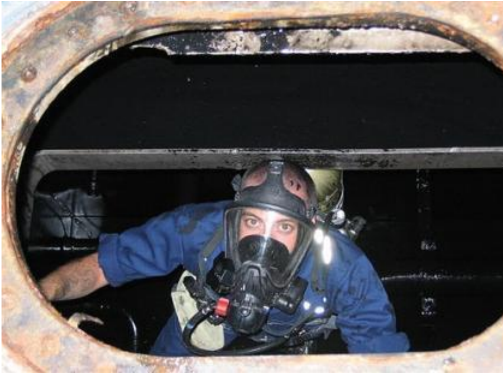
Fig. 15.1 A: Entering enclosed space with SCBA
