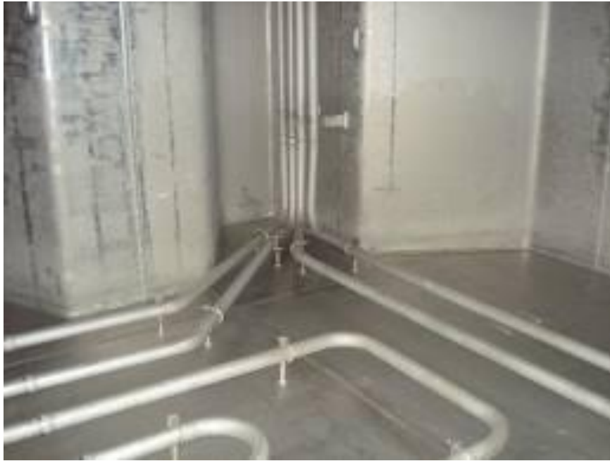
Fig. 1.8 G: Heating arrangements of a Chemical Tanker
