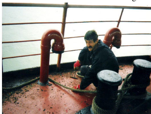
Figure 28 Maintenance of the deck
