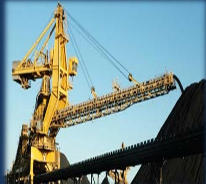
Pic.12 Stockyard Reclaimer Crane
