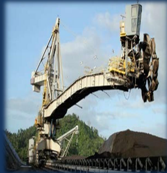
Pic.10 Bucket-wheel Stacker/Reclaimer
