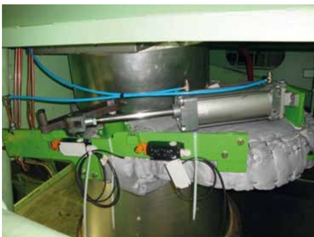
Fig. 28: T/C cut-out valve (compressor side)
